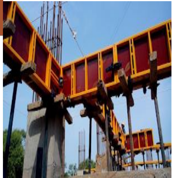
Beam Shuttering
